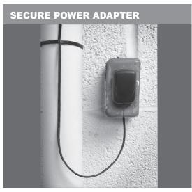
**4.** Plug the power adapter into a protected indoor or outdoor outlet, leaving enough slack for a "drip-loop," preventing rain water from trailing into the outlet. Installation is complete.
